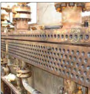
FinFan cooler before a maintenance
