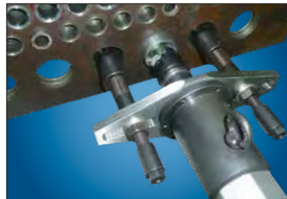
Reducing tube wall on a 6" thick tube sheet prior to punching.
